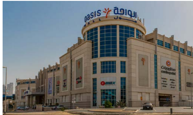
Project name: Renovation of Oasis Mall for Landmark Group
