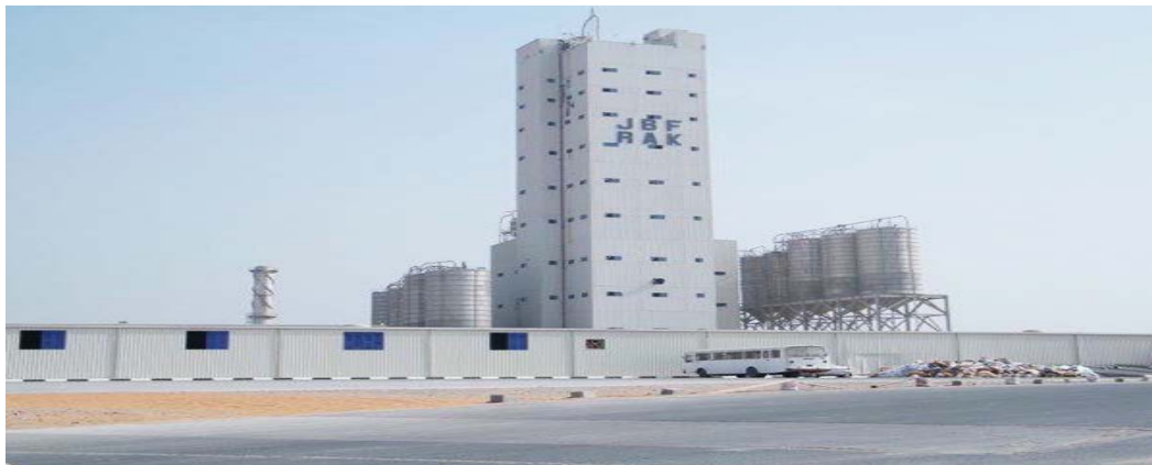
Project name: Plasma Screen plant for JBF Group
